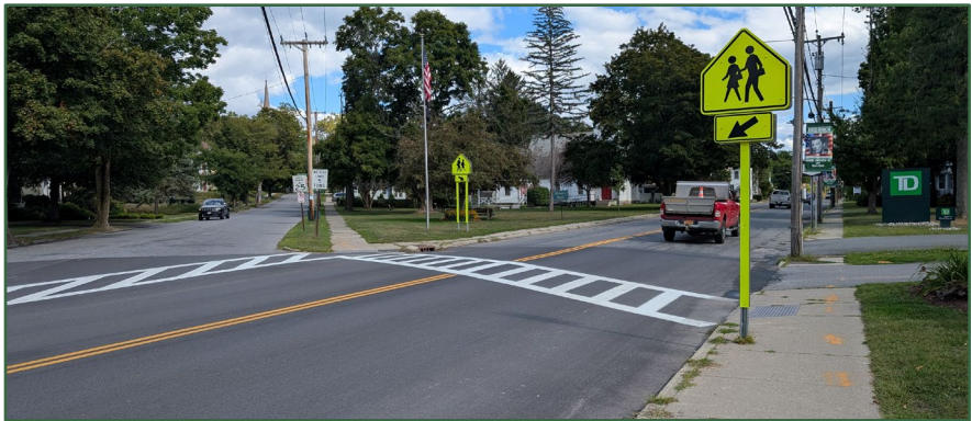
Above: Existing sidewalk condition
