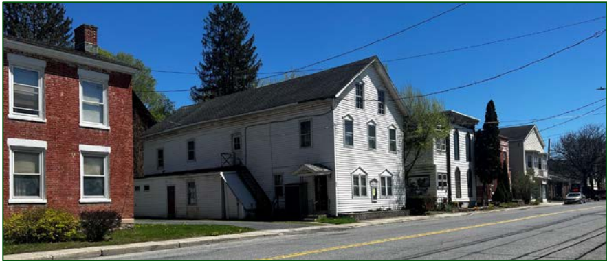
Above: Existing site exterior
