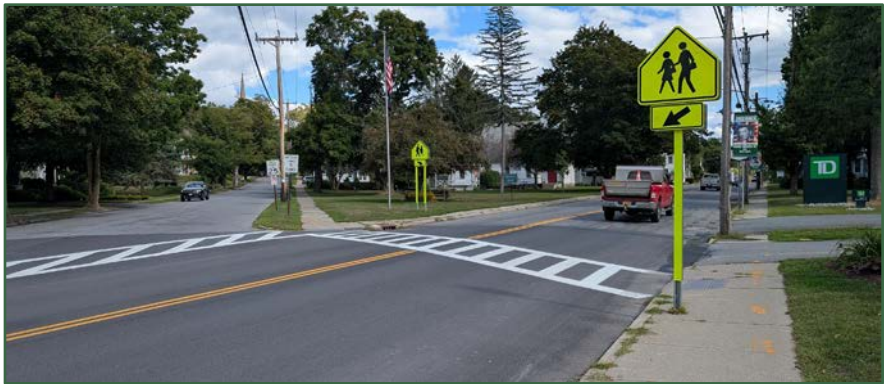
Above: Existing sidewalk condition
